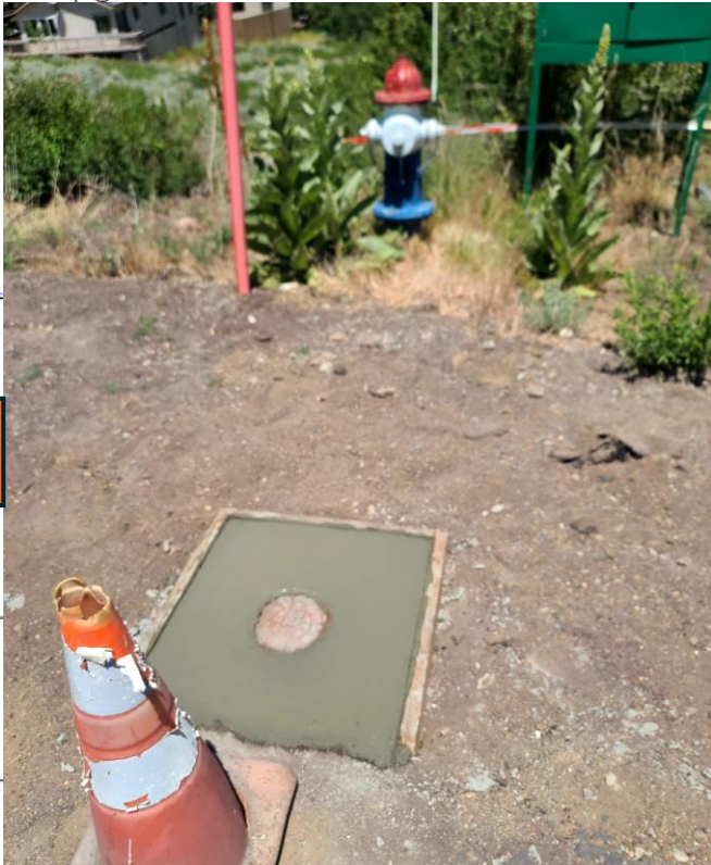
Broken standpipe repaired and protected by a concrete apron
